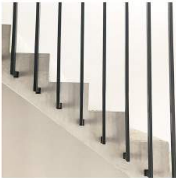
Directly installation on staircase
